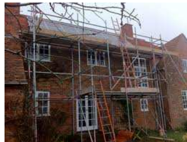
Local scaffold companies x 5
